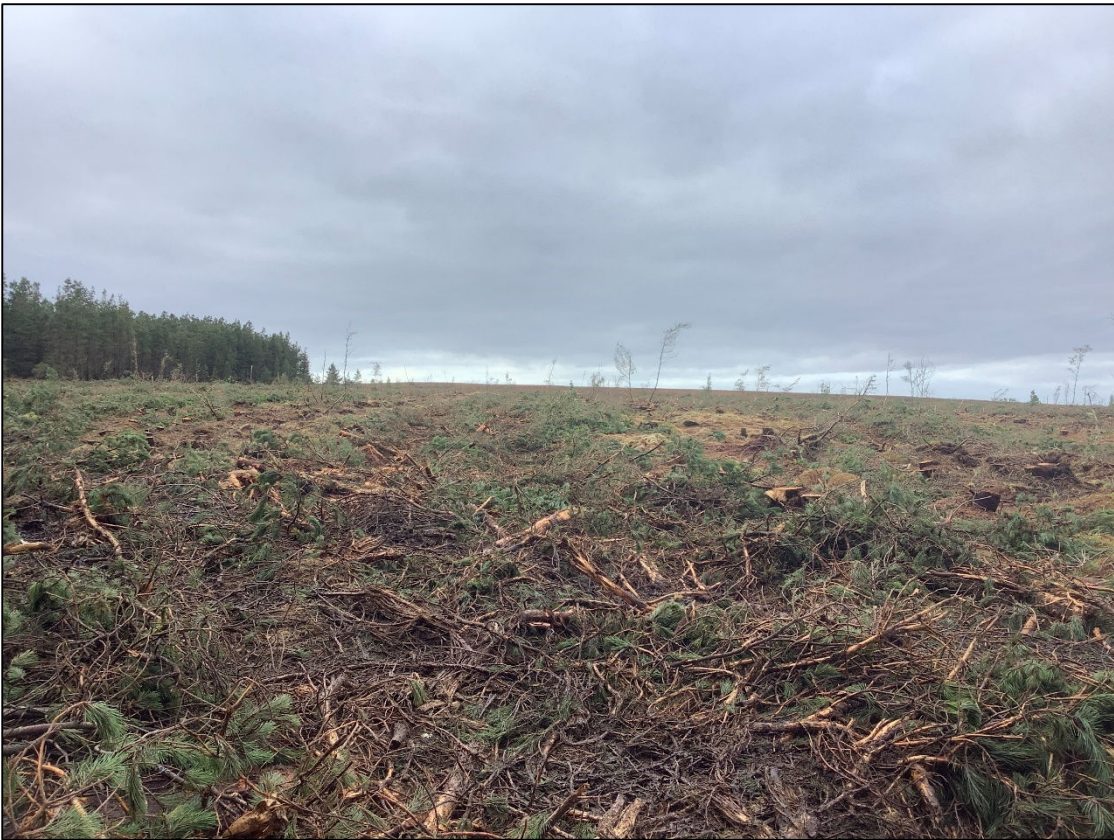
Plate 13-5: Area of proposed turbine 2 looking West.
