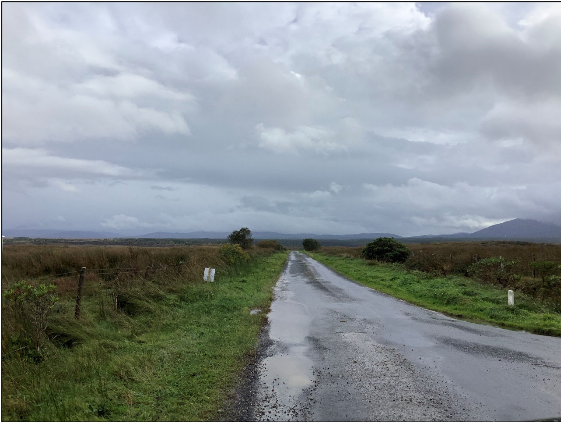
Plate 13-51: Proposed grid connection route looking south.
